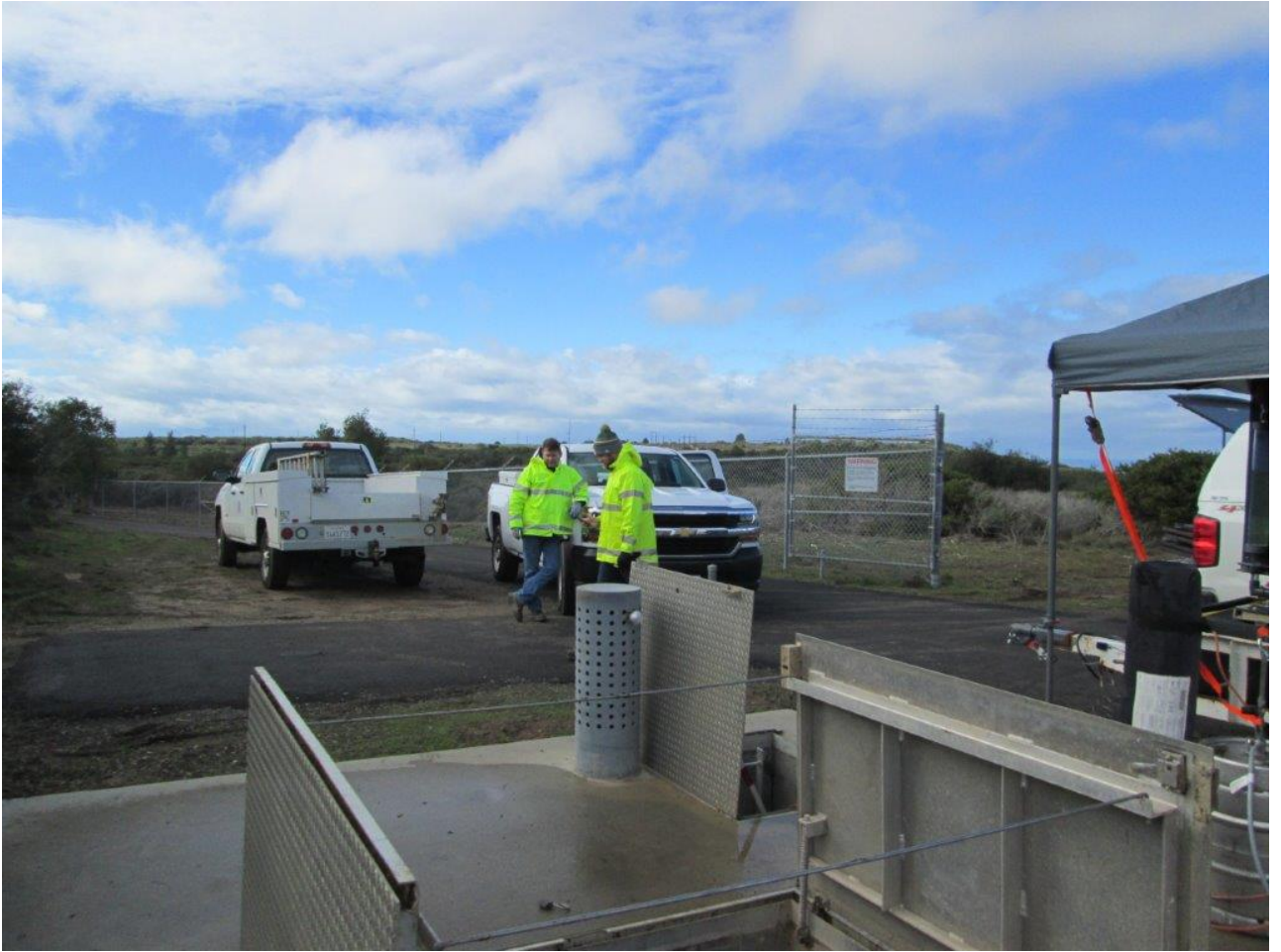
Tank 5 Inlet Vault, February 2022
