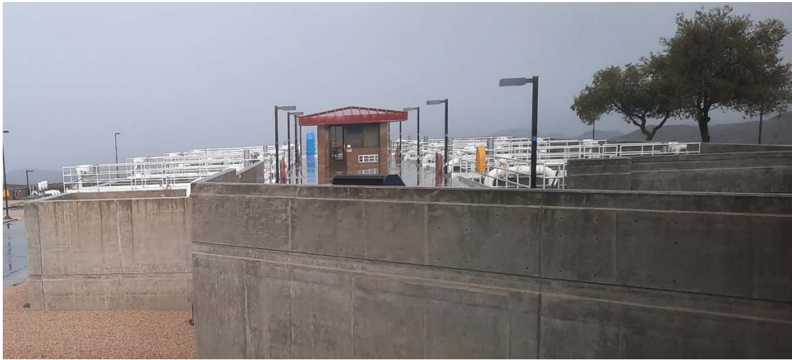
Water Treatment Plant February 2022
