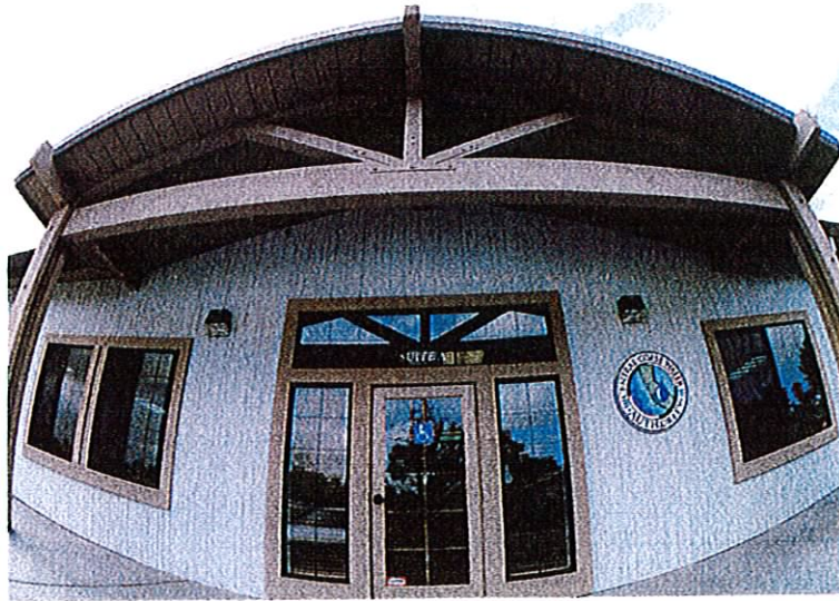
The Central Coast Water Authority Administrative Office. The Authority leased the office effective August 1, 1994, moved into it on October 3, 1994 and subsequently purchased it on December 1, 1998.
