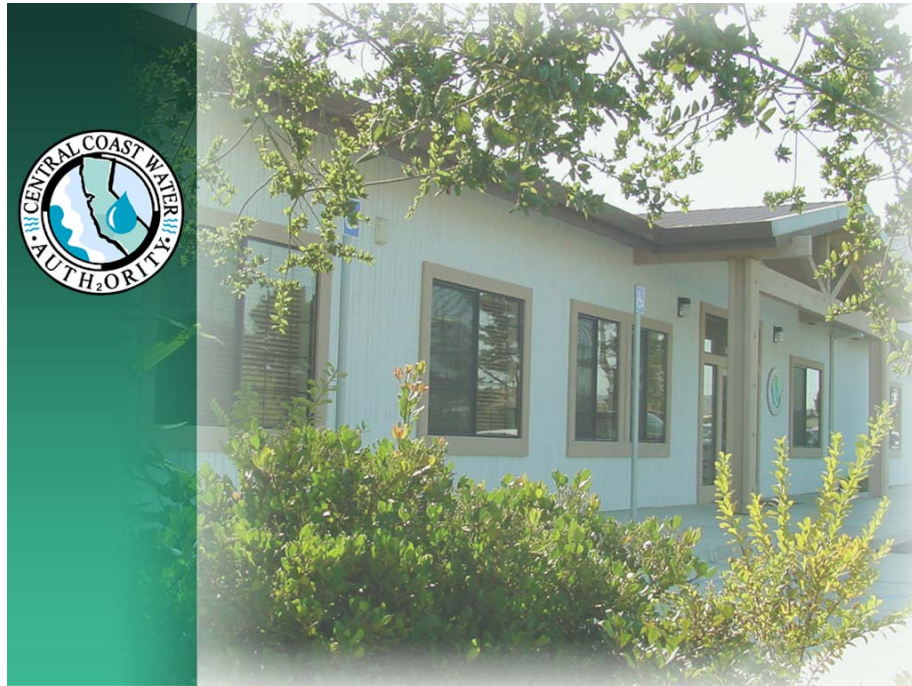
The Central Coast Water Authority Administrative office. CCWA leased the office effective August 1, 1994, moved into it October 3, 1994 and subsequently purchased it on December 1, 1998.
