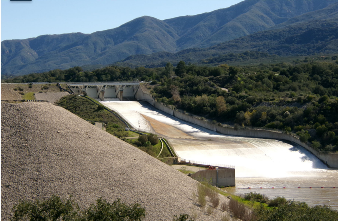
Bradbury Dam Spillway March 2023
