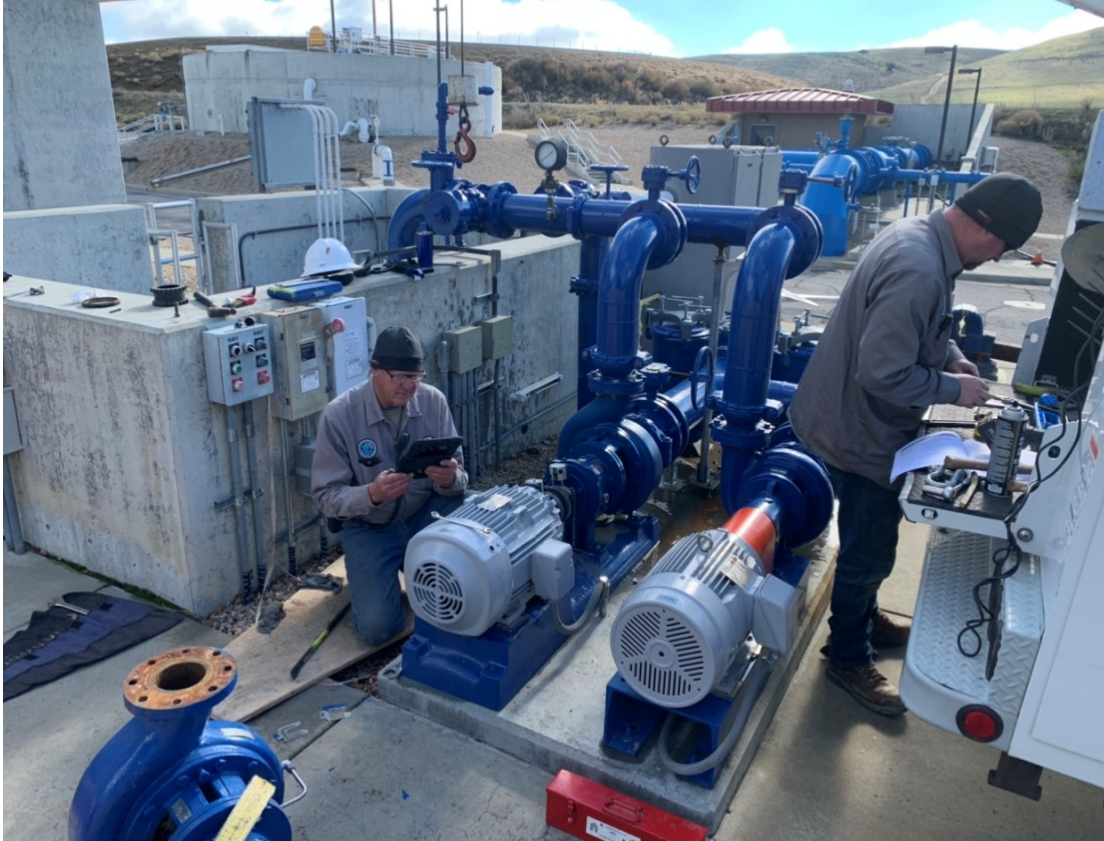
Flash Mix Pump Install January 2023
