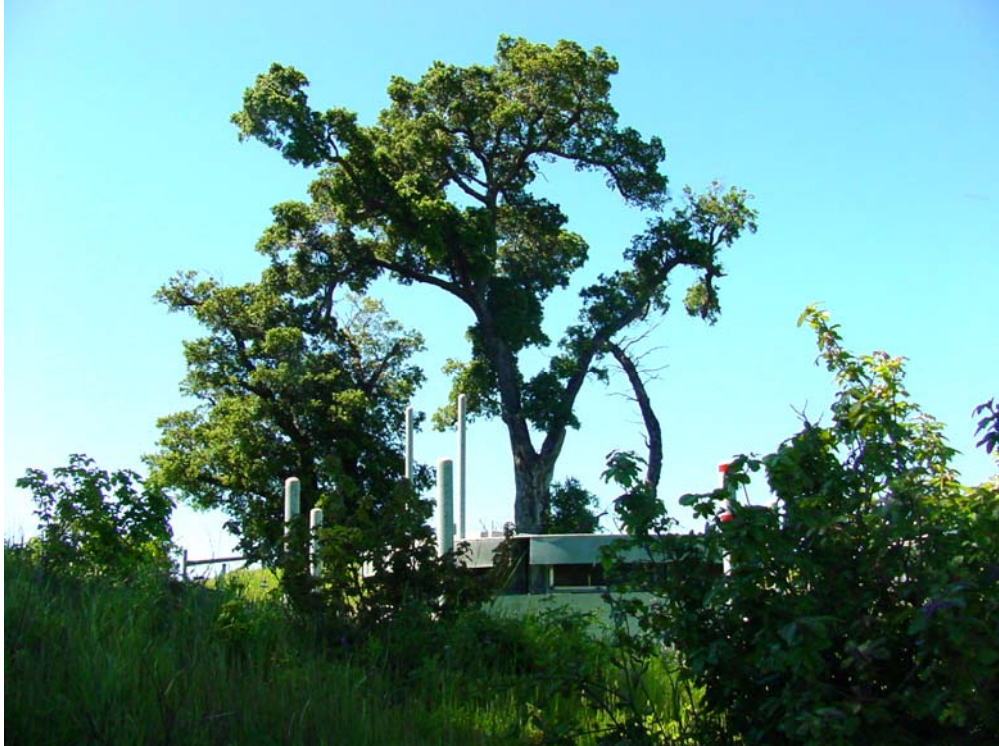
Santa Margarita Ranch Air Vacuum/Air Release Vault (Power Line Hill).
