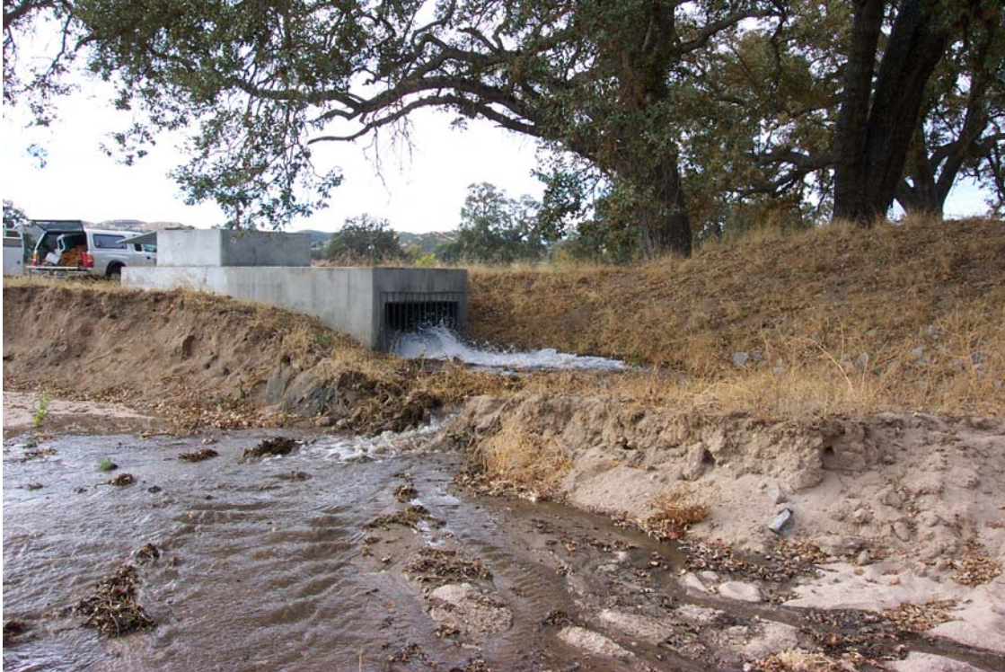
Dewatering structure on the east branch of the Huerhuero Creek.
