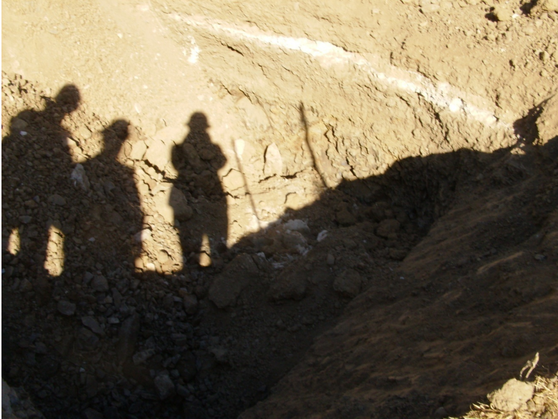
Staff observing work in the right-of-way
