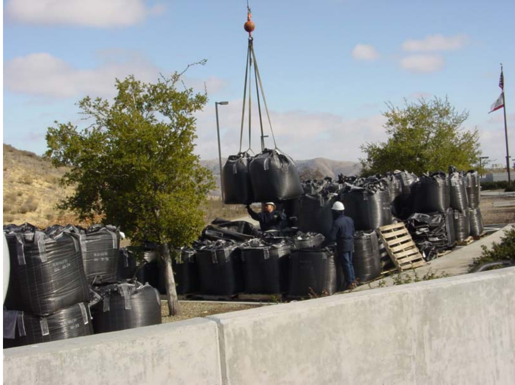
Granular activated carbon for replacement in filters at Polonio Pass Water Treatment Plant
