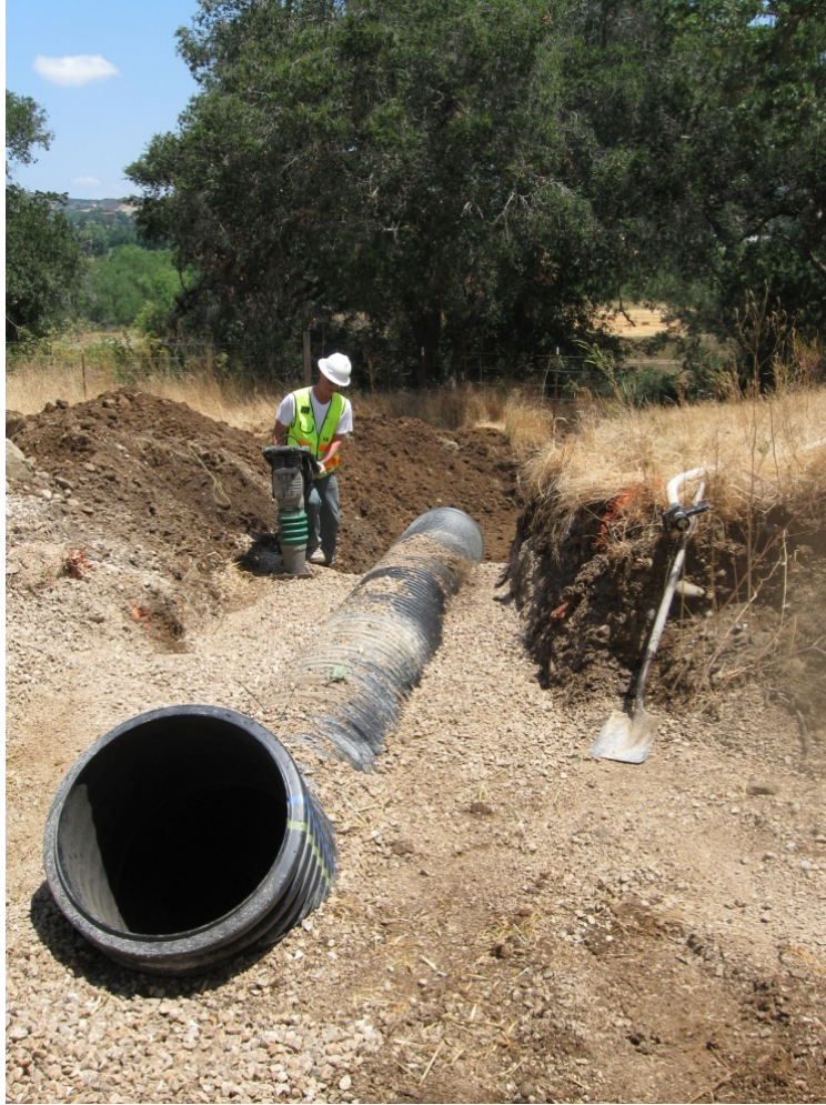
Erosion repair on the pipeline near Buellton
