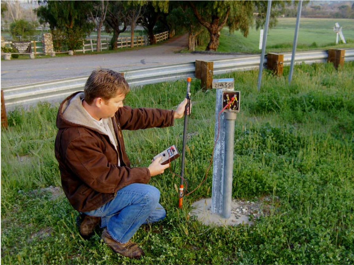
Conducting cathodic protection system survey near Santa Ynez
