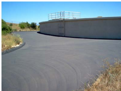
Slurry seal of Tank 5 pavement
