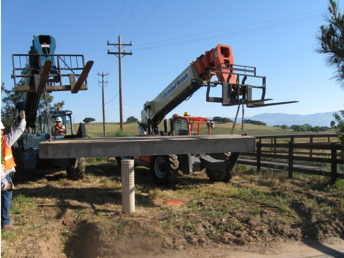
Santa Ynez Pumping Facility Outlet Vault Lid Replacement
