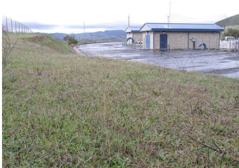
Energy Dissipation Vault
