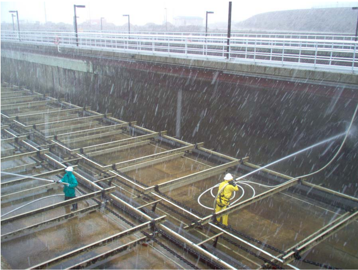
Sedimentation basin cleaning at Polonio Pass Water Treatment Plant
