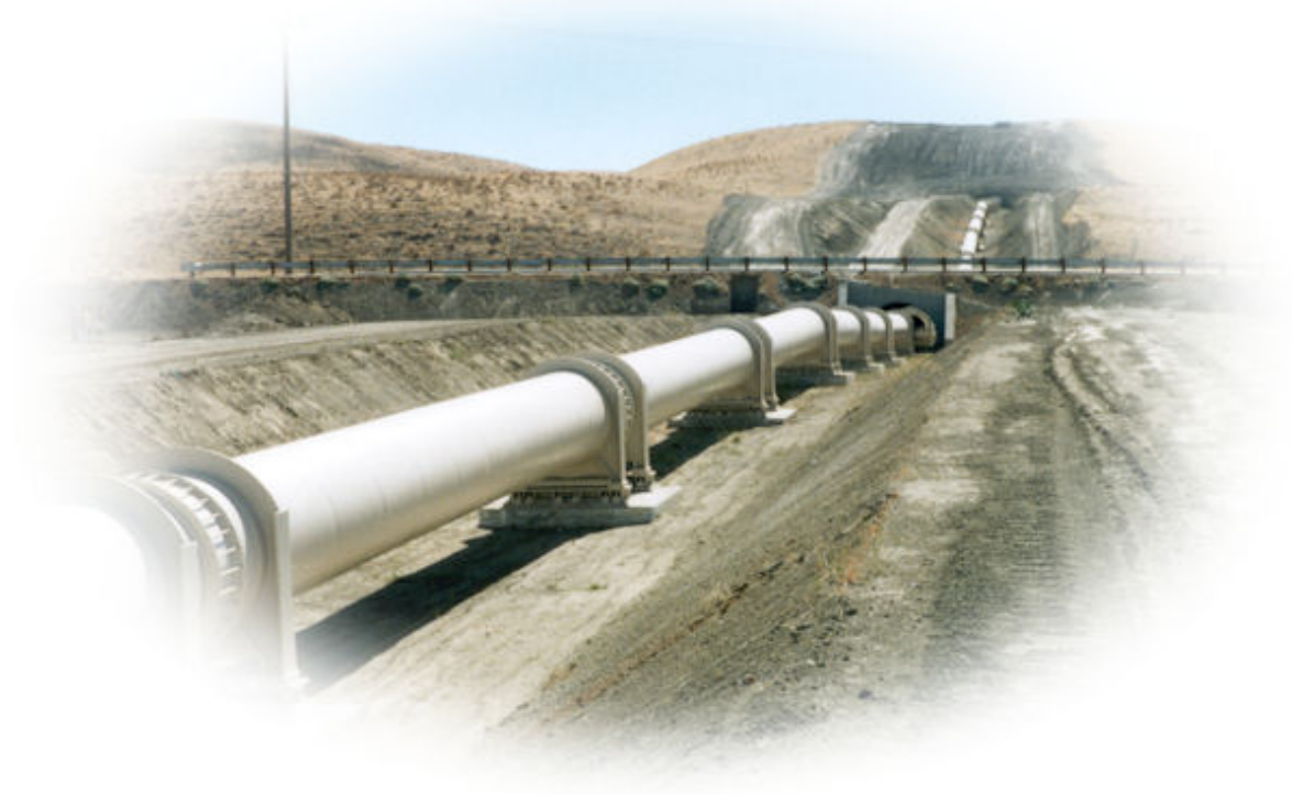
Pipeline crossing San Andreas Fault
