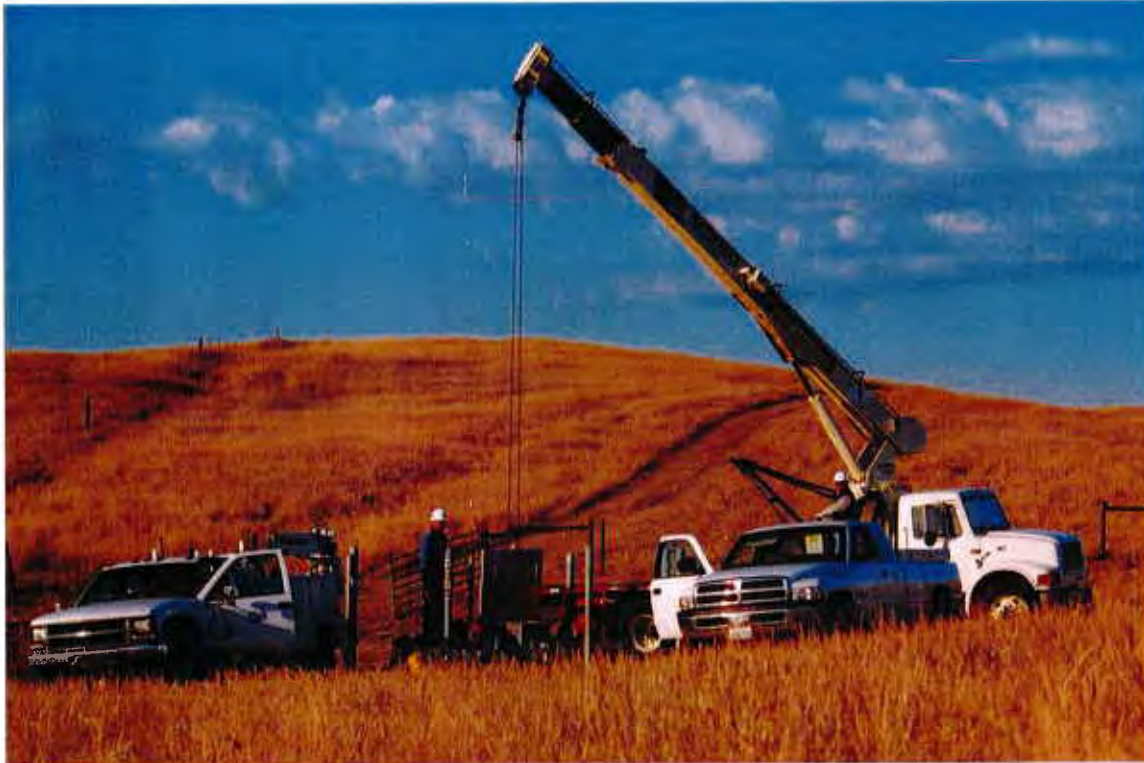
CCWA staff removing vault lid during Reach 2 inspection, November 2003.
