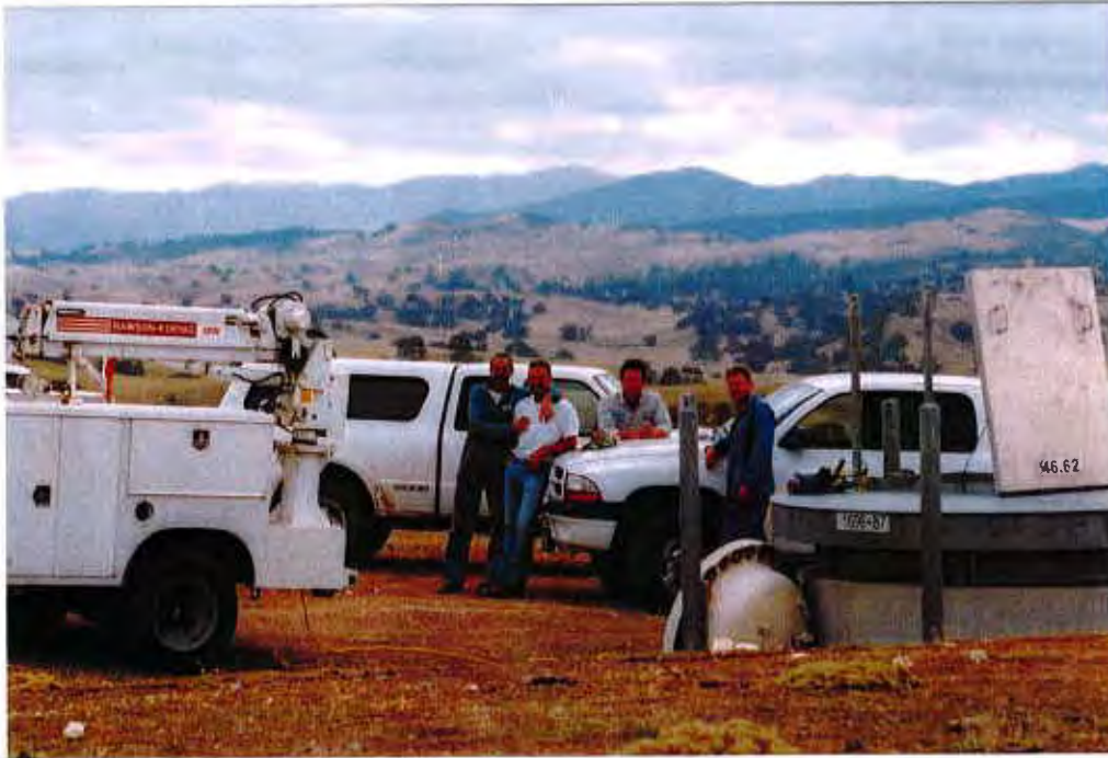
Reach 2 inspection, November 2003, CCWA staff regroups after assessment of the pipeline interior.
