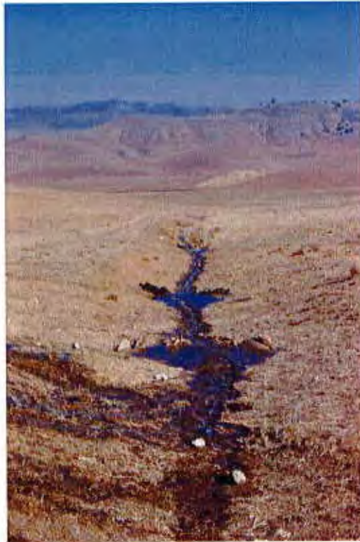
Pipeline dewatering near Chalome prior to the November 2003 pipeline inspection.
