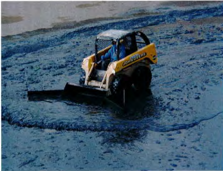
Clay/silt removal from Polonio Pass raw water tanks..
