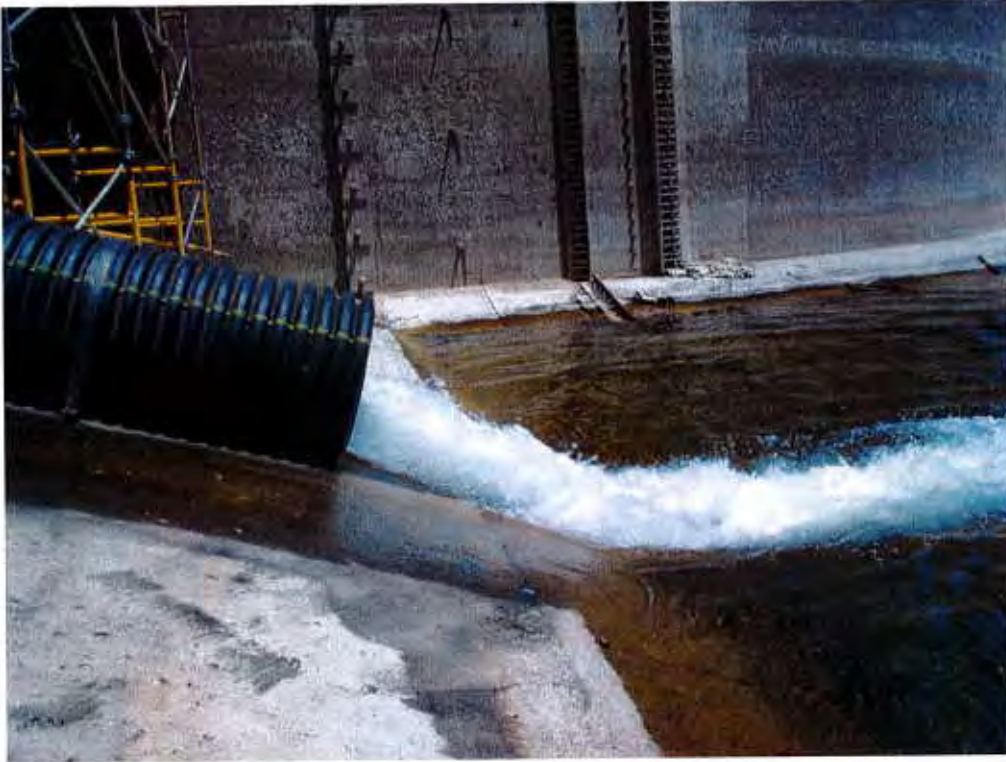
Temporary State Water Project pipeline delivering State water for the South Coast project participants into Lake Cachuma.
