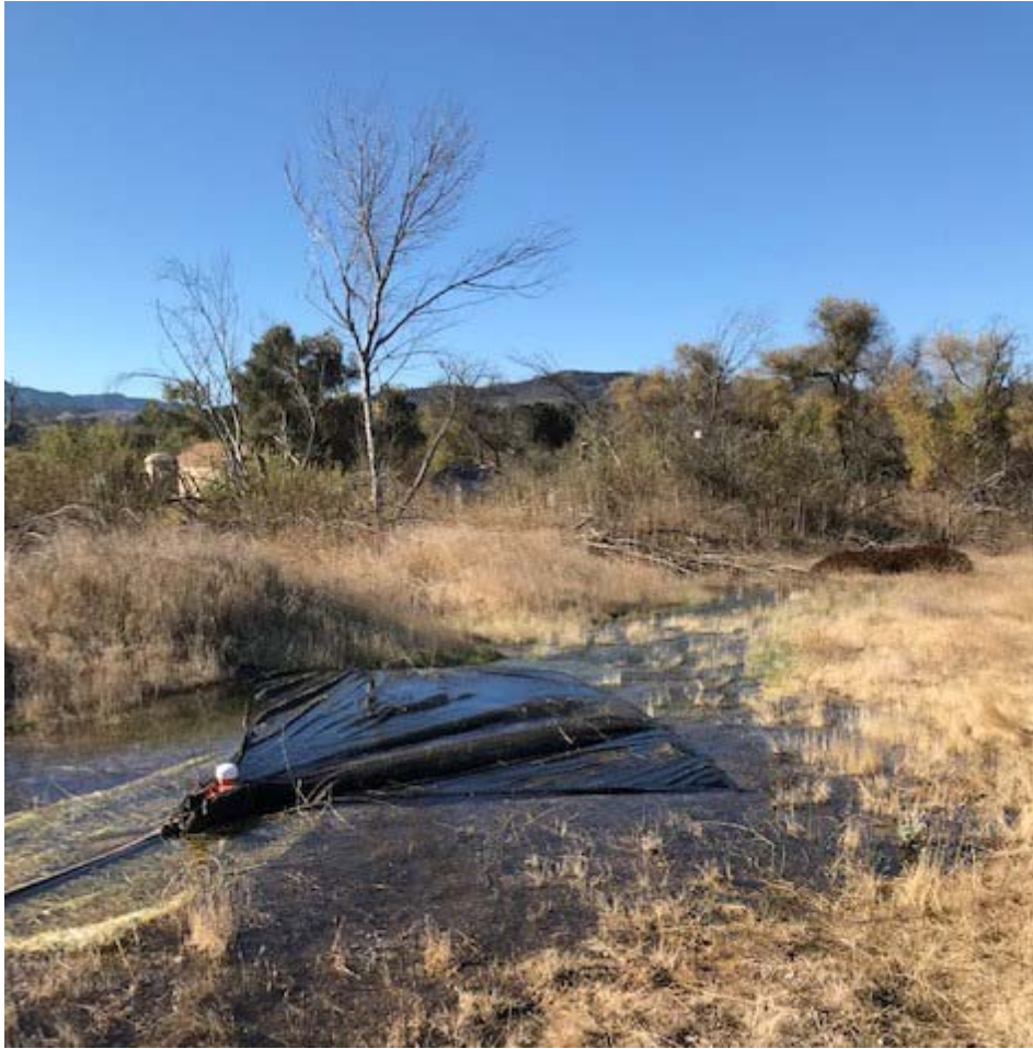
Dewatering site below the Santa Ynez Mission prior to Winter Shutdown 2019
