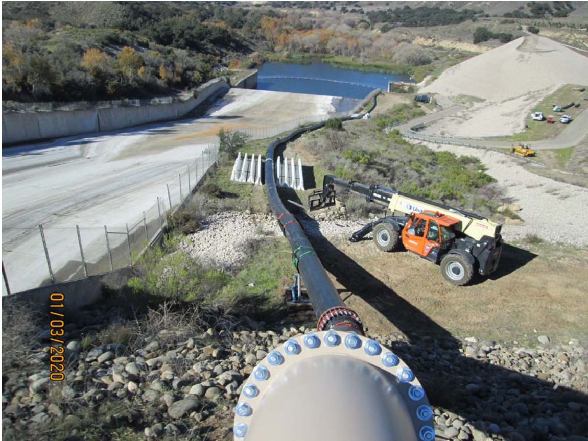
Bypass Pipeline Installation at Bradbury Dam January 2020
