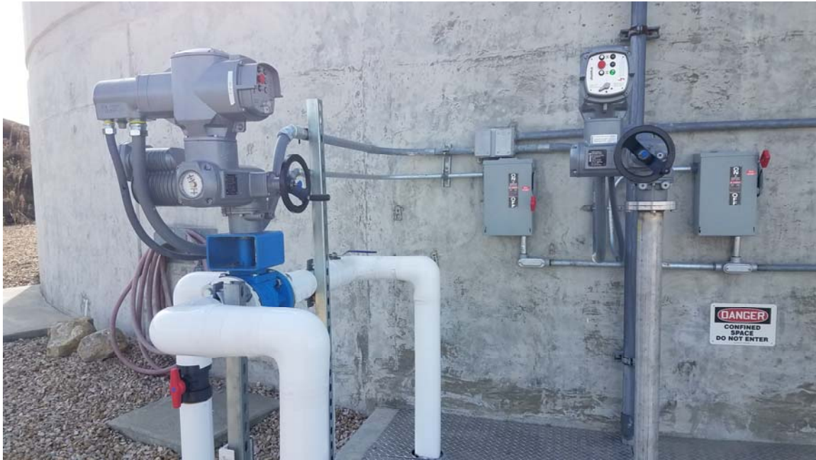
Water Treatment Plant Clarifier Valve Replacement 2019
