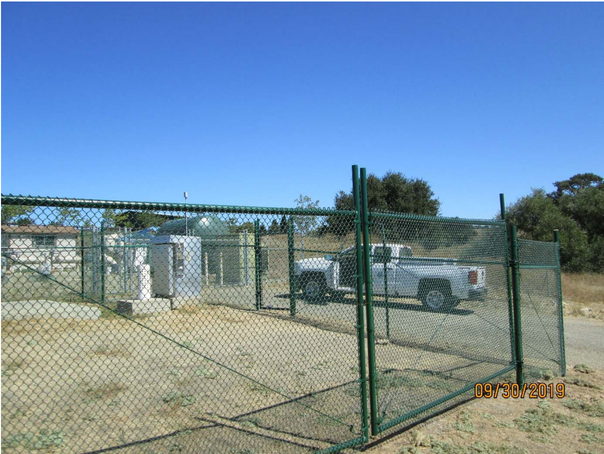
Facility Fencing Project prior to completion September 2019
