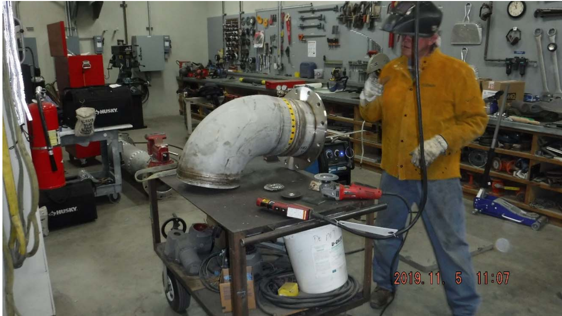
Polonio Pass Water Treatment Plant Air Scour Valve Replacement Project November 2019
