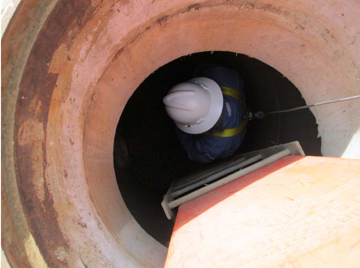
Staff accessing vault for inspection 2019
