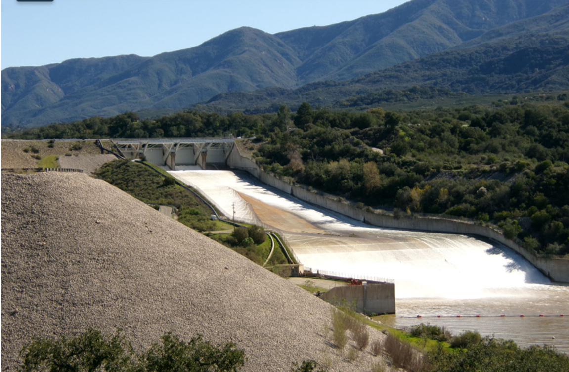
Bradbury Dam Spillway March 2023
