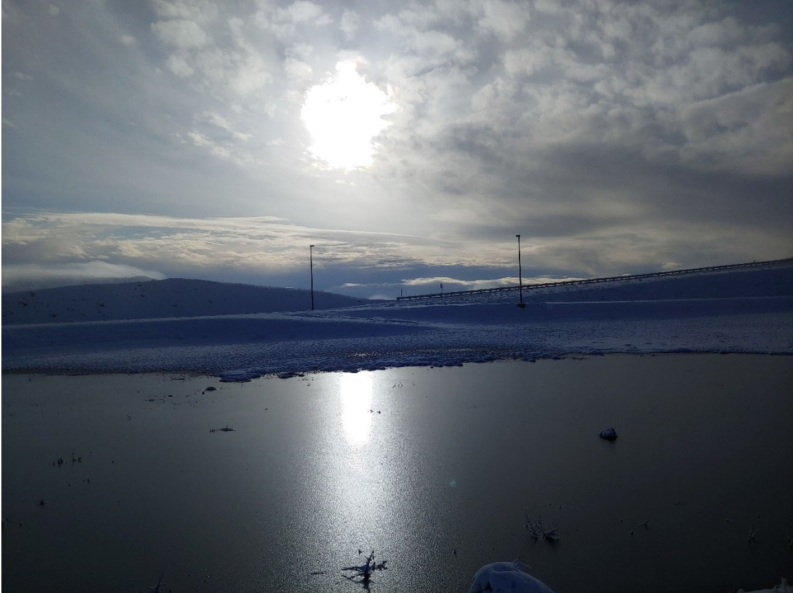
Water Treatment Plant Snowstorm 2023
