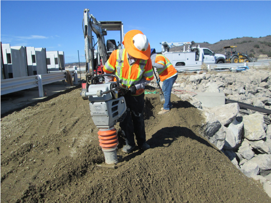
Cachuma Lake Pipe Extension Project 2023
