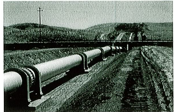
Pipeline crossing the San Andreas Fault four miles downstream of the treatment plant. The pipeline is not buried for this crossing and each section of pipe is connected with a flexible joint.
