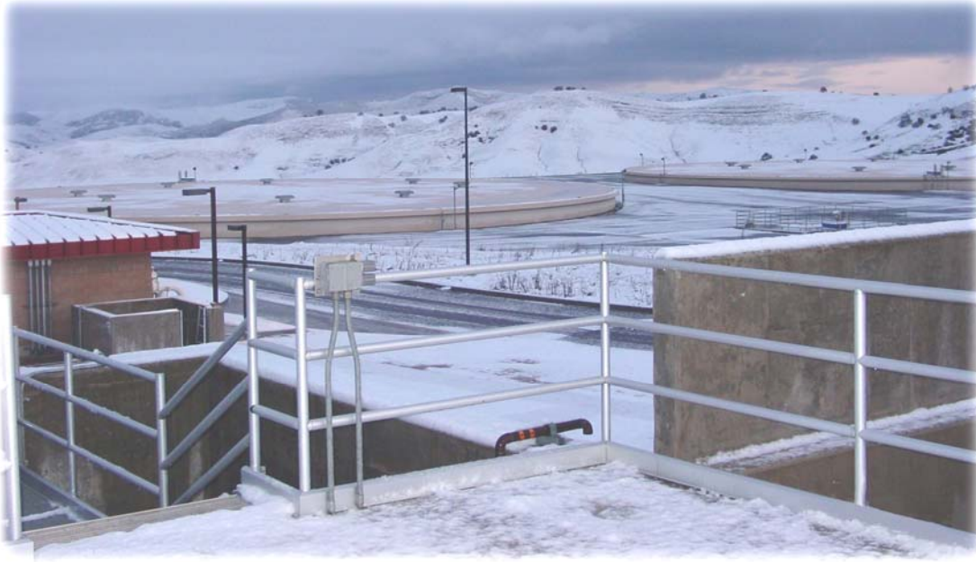
Winter, Polonio Pass Water Treatment Plant
