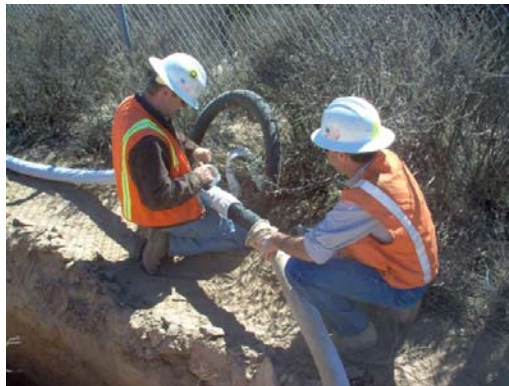
Installation of drain line
