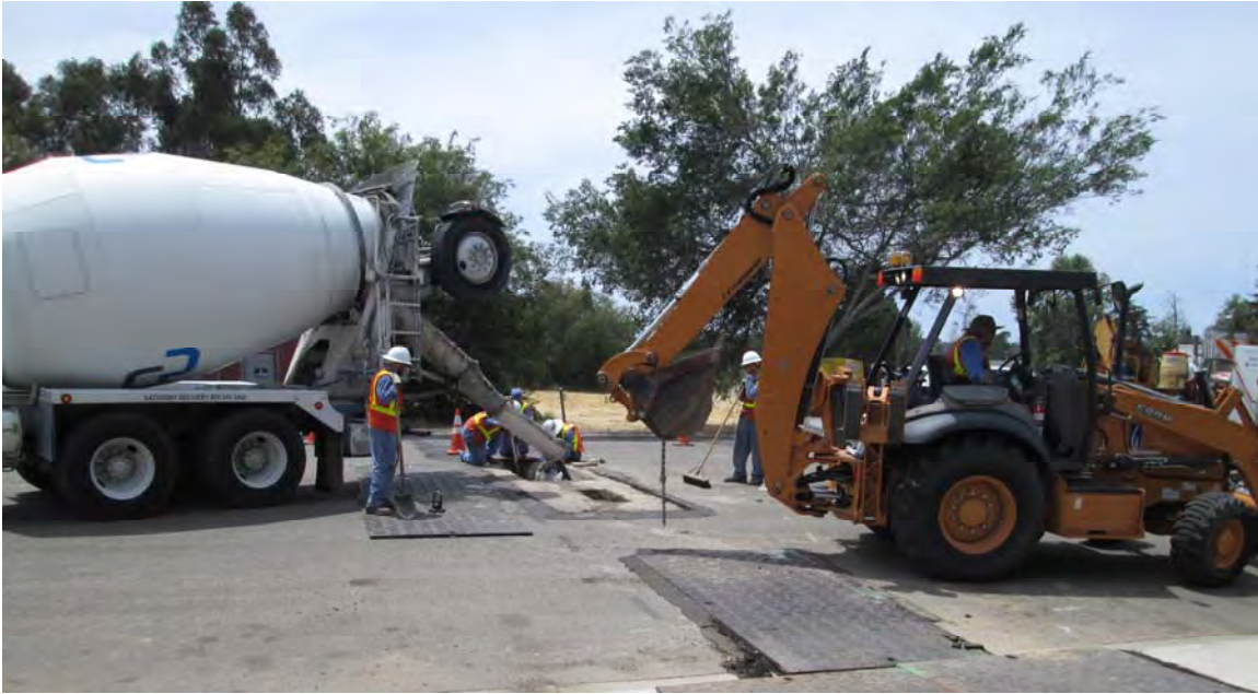
Thompson Avenue, Nipomo - Void Repair
