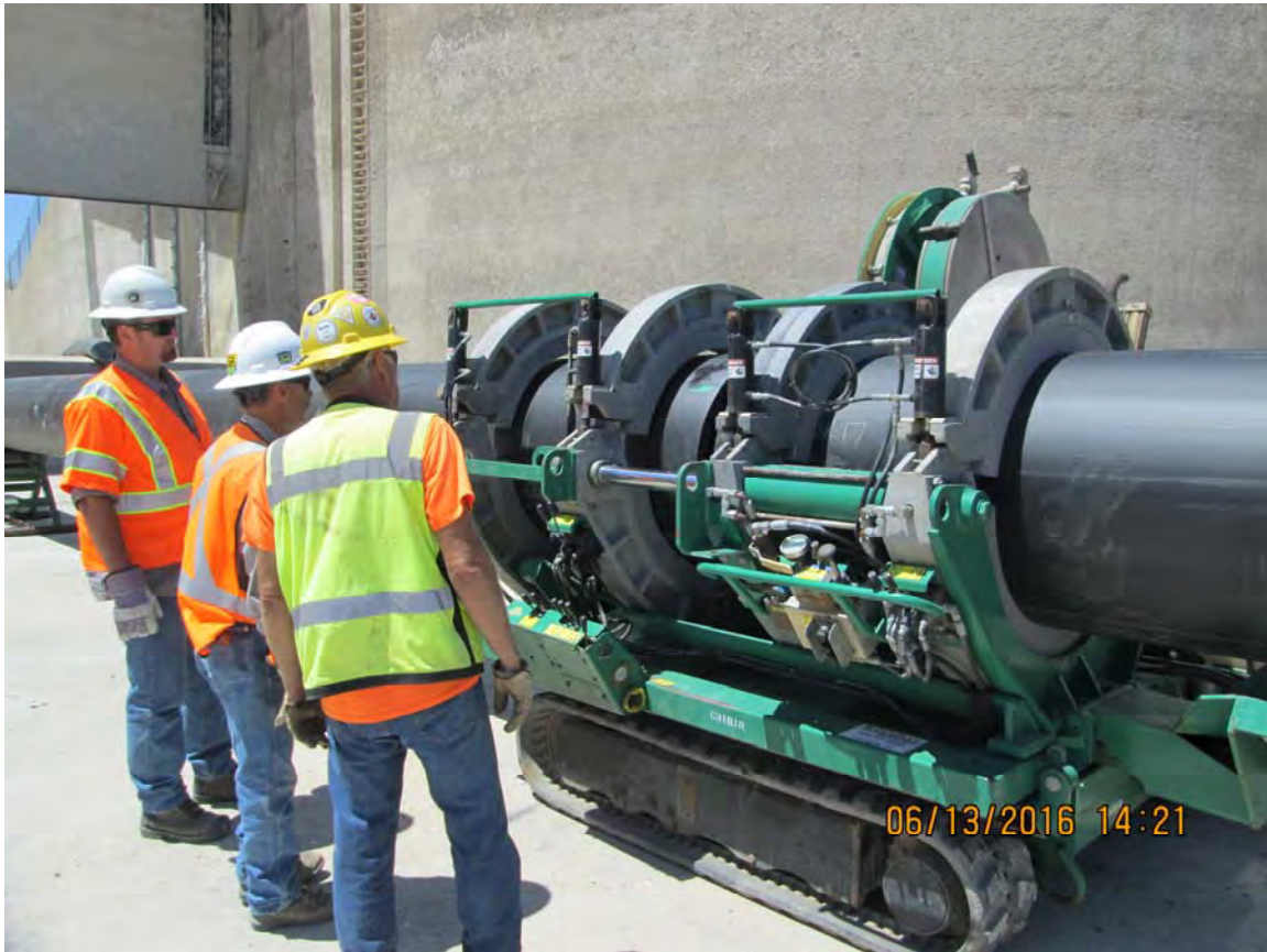
Bypass Pipeline Assembly at Bradbury Dam
