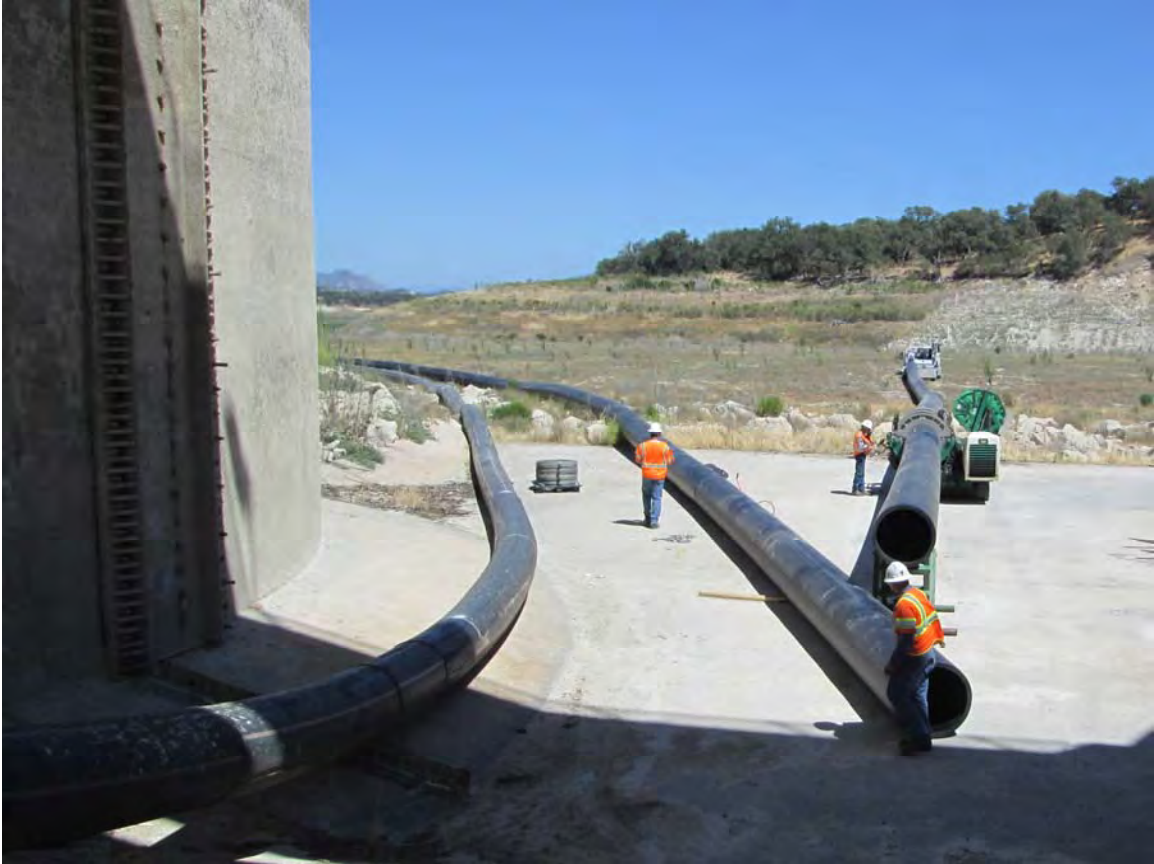
Assembly of Bypass Piping at Bradbury Dam
