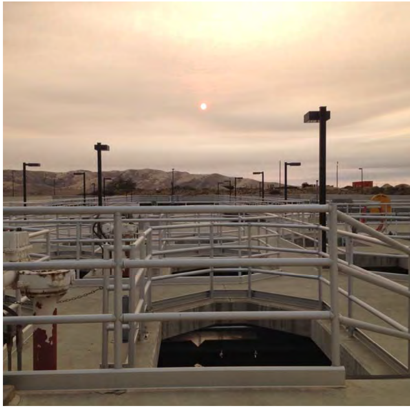
Water Treatment Plant sunset (September 2015)
