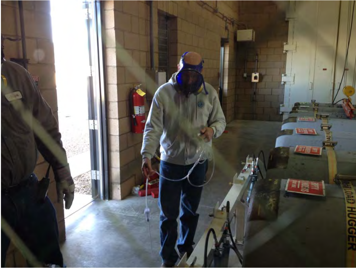
Air Quality Testing During Chlorine Header Replacement Project
