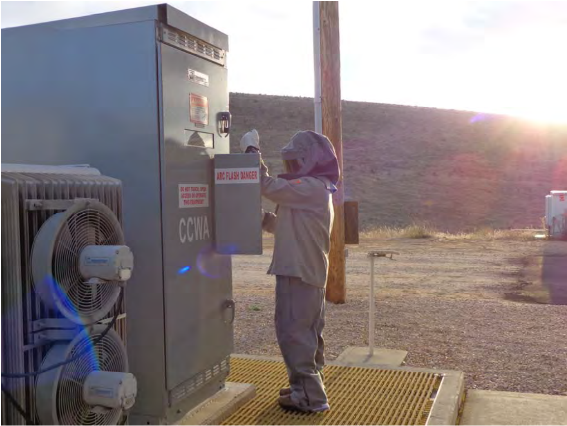
Arc Flash Safety Gear in Use During Circuit Opening
