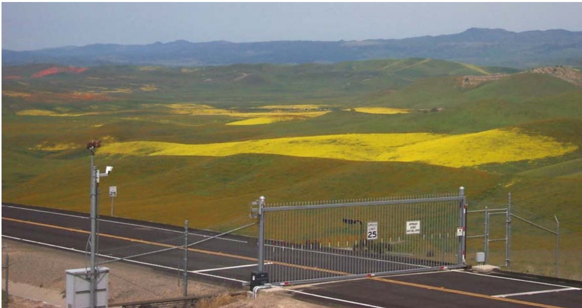
Polonio Pass Water Treatment Plant Gate
