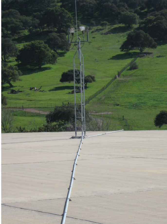
Security Cameras at Tank 7
