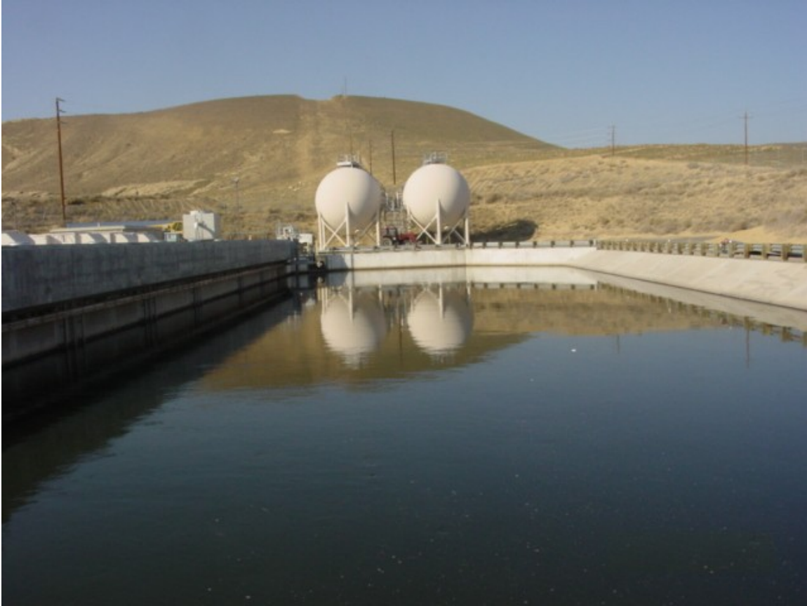
Forebay at Devils Den Pump Station
