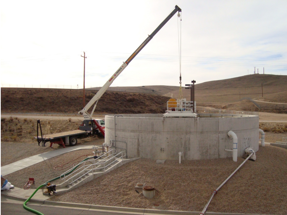
Clarifier Turbine Repair
