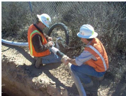
Installation of drain line
