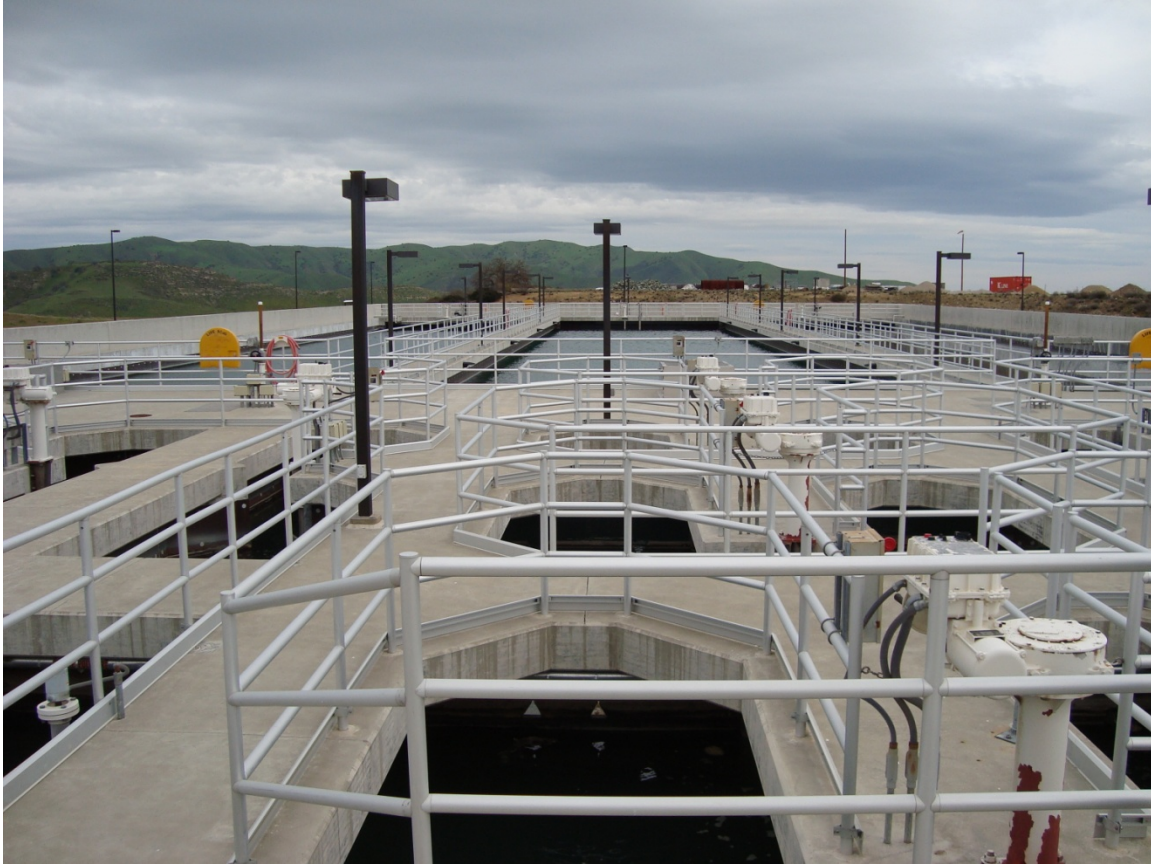
Flocculation and sedimentation basins
