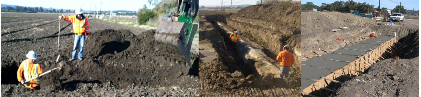
La Purisima Roundabout Encasement Project
