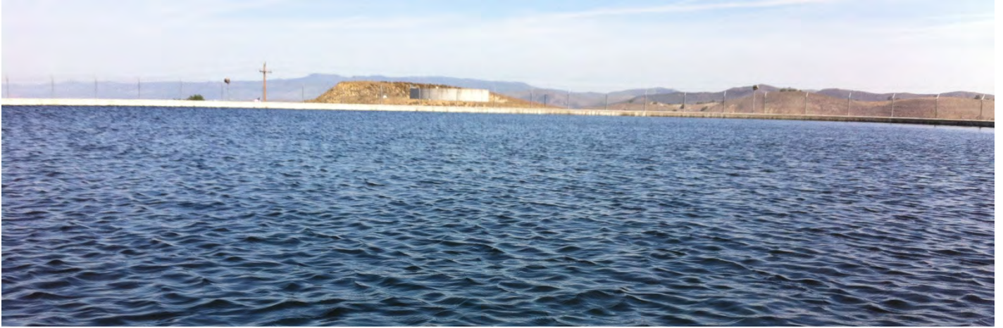
DWR Raw Water Tank 3 approximately 10" from spilling on April 16, 2012
