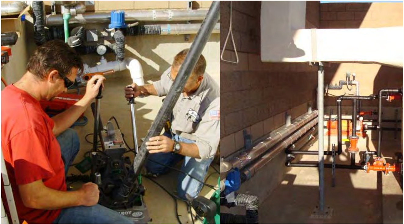
Chlorine Scrubber Caustic Pump Re-pipe Project
