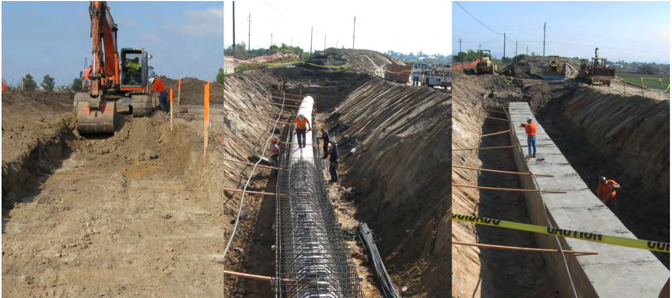
Willow Road Encasement Project - December 2011
