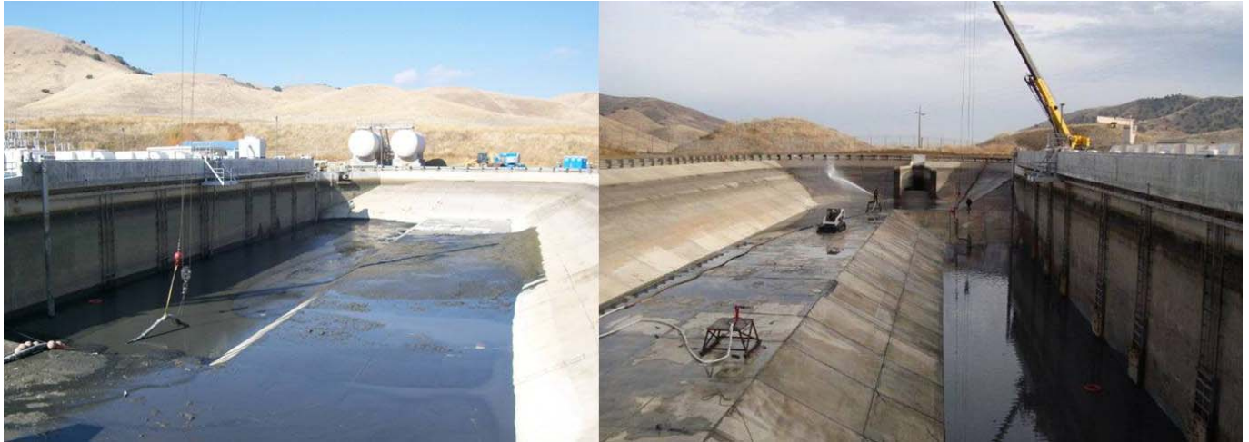
Polonio Pass Pumping Plant Forebay Sediment Removal
