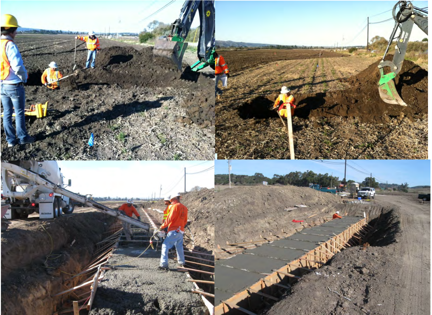
La Purisima Roundabout Project - December 2011
