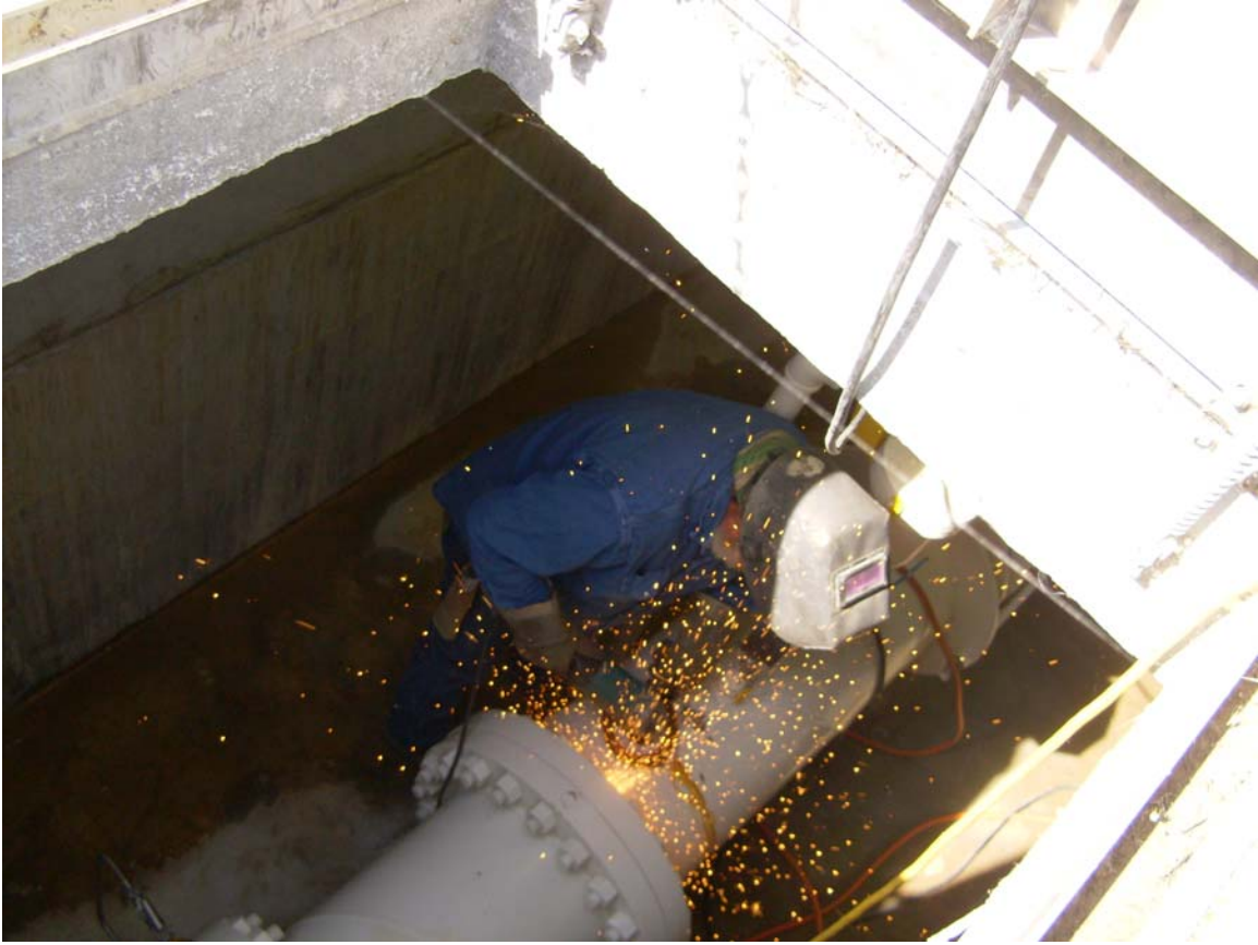
Chorro Meter Vault Leak Repair
