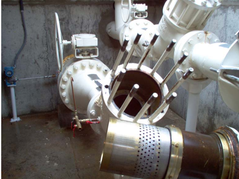
Chorro Turnout Sleeve Valve
