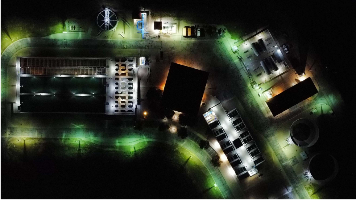
Polonio Pass Water Treatment Plant at night
