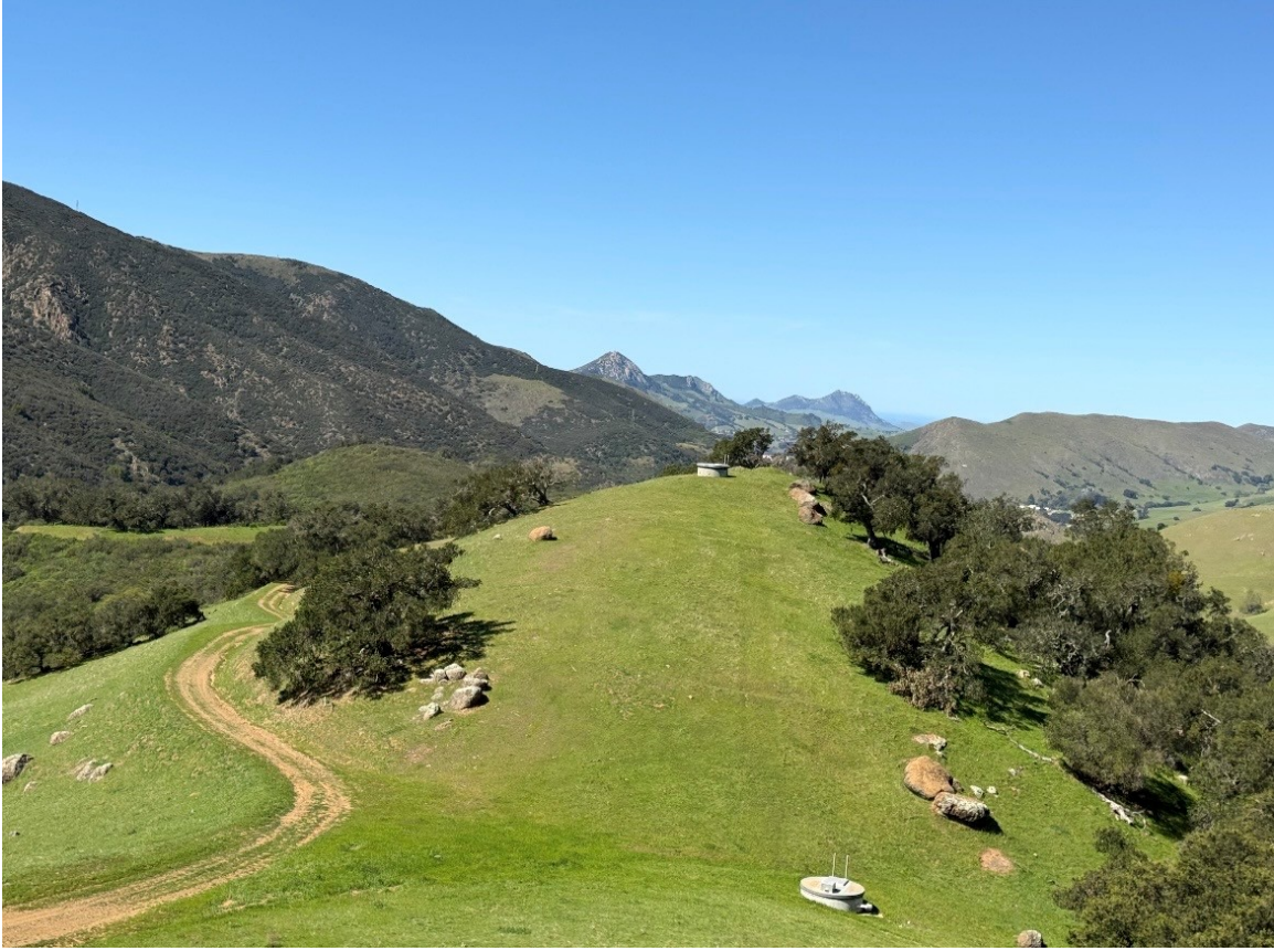
Air vac vaults at Reservoir Canyon in San Luis Obispo County
