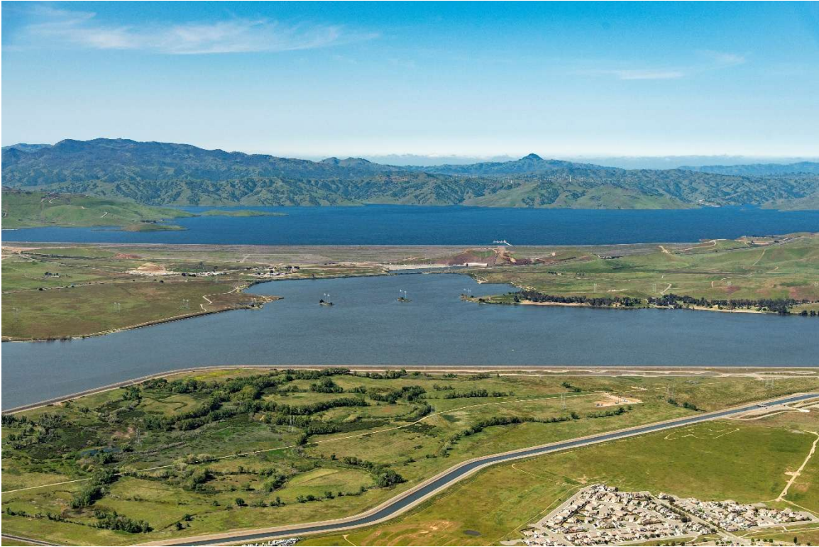
Delta-Mendota Canal and O'Neill Forebay in the foreground, San Luis Reservoir near Los Banos in background (Photo Courtesy of DWR)
