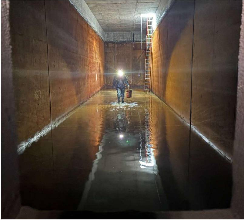
Inspecting Chlorine Contact Basin during annual maintenance shutdown
