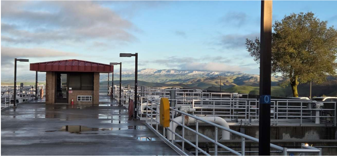
Polonio Pass Water Treatment Plant
