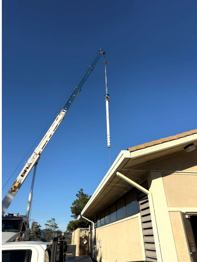
Pump being removed for repair at Santa Ynez Pumping Plant
