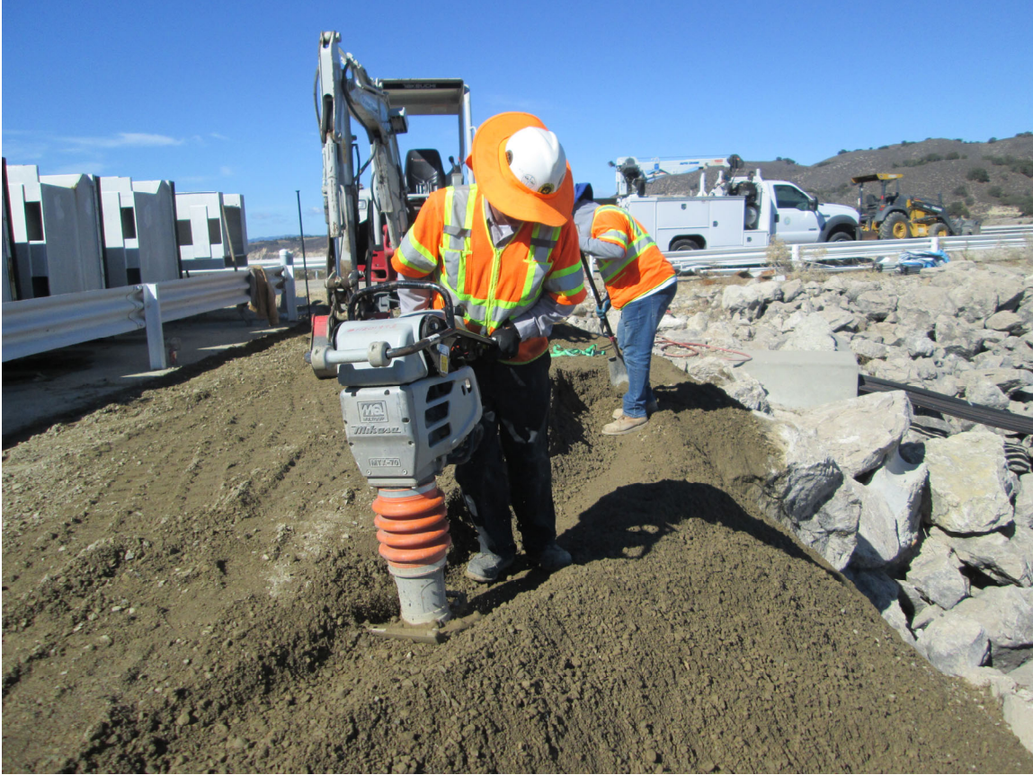
Cachuma Lake Pipe Extension Project 2023
