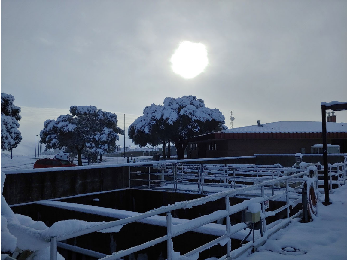
Water Treatment Plant March 2023
